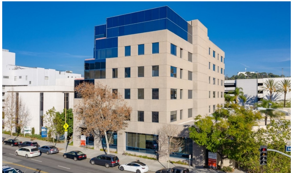
The six-story, 67,060-square-foot Glendale MOB II in Glendale, Calif., is 89 percent occupied with a diverse mix of healthcare provider tenants.
